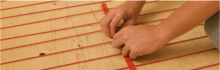
FIGURE 2.29: Install stabilizing guides
