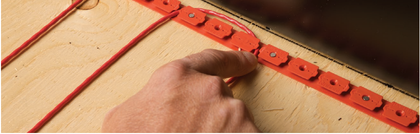
FIGURE 2.26 : Installer le câble chauffant
