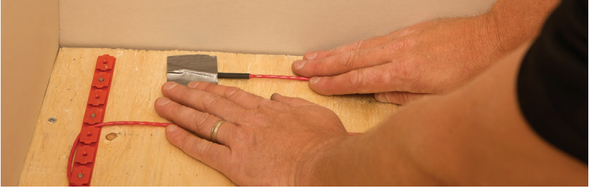
FIGURE 2.28: Secure the end seal
