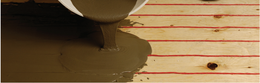
FIGURE 2.42: Self-leveling compound method
