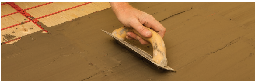
FIGURE 2.52: Thinset mortar method
