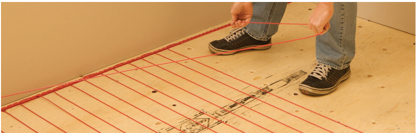
FIGURE 2.27 : Installer le câble chauffant
