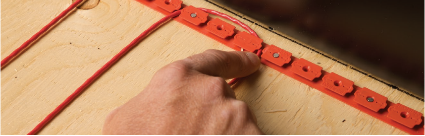
FIGURE 2.26: Install the heating cable
