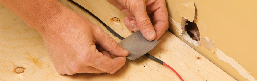
FIGURE 2.23: Secure the cold lead to the subfloor
