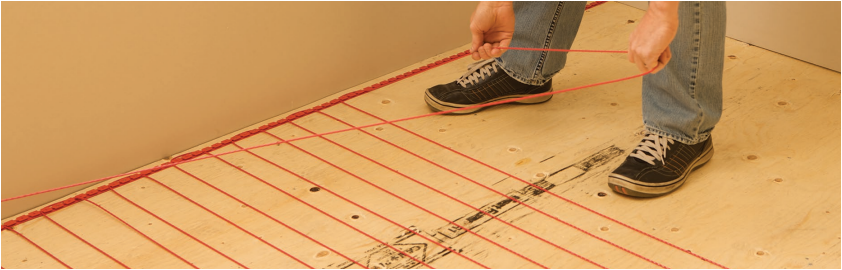
FIGURE 2.27: Install the heating cable
