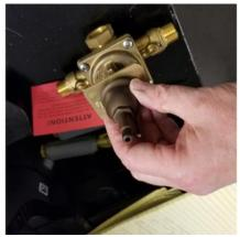
5. Position #3 wall plate over #2 mounting plate center post. Make sure you align it with the "Herbeau France" lettering at the top and Froid (cold) and Chaud (hot) are aligned with the cold and hot rough inlets. Thread #13 locking nut over center post and tighten with adjustable wrench so wall plate is secure:
